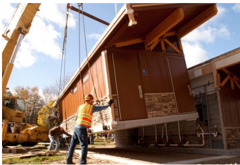
Workers put restroom module in place at Nicolet Beach
